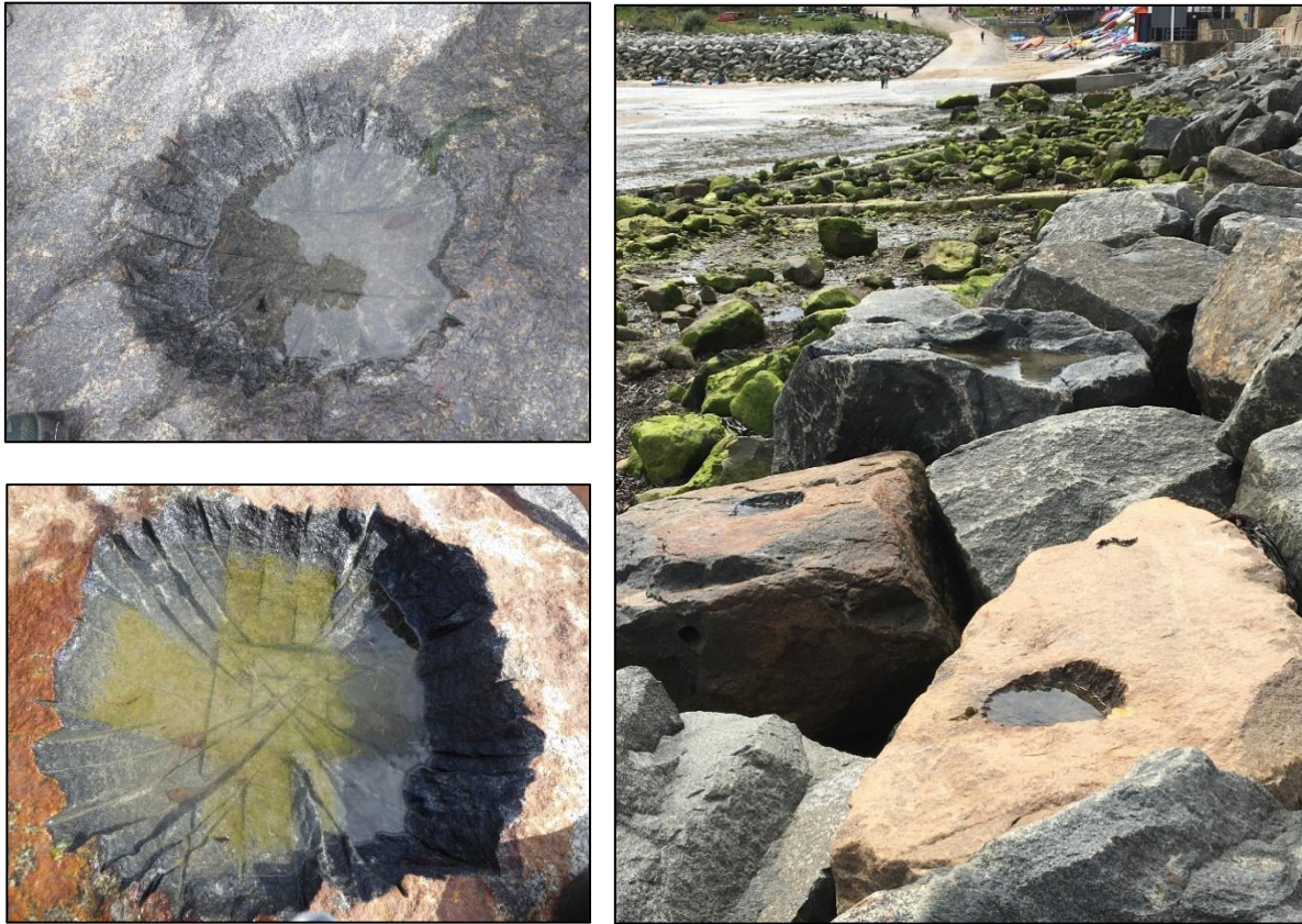
Figure 2.2. Examples of saw cut artificial rock pools roughly 300 mm diameter x 150 mm deep.
